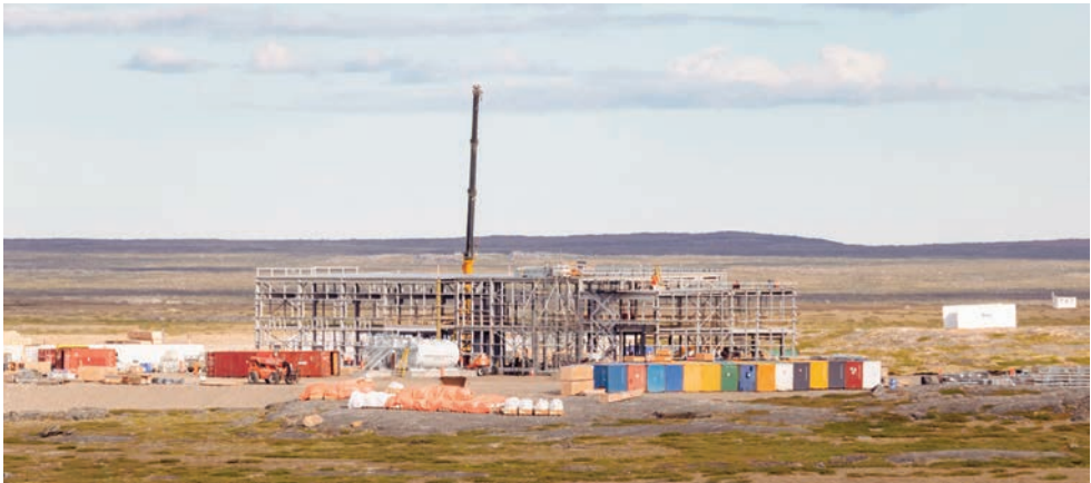
Aupaluk’s new power plant, currently under construction, is scheduled to start producing power in 2027. (Photo by Jeff Pelletier)
