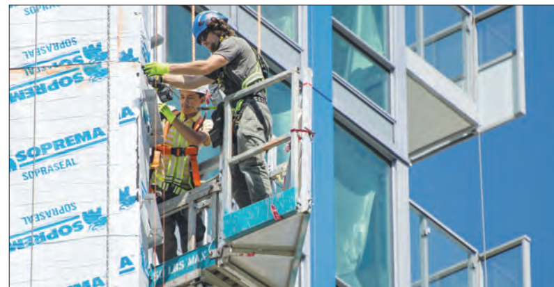
Workers on a platform attach a piece of construction material to a new building at the Apex at Seylynn Village development in June 2023. NICK LABA / NSN FILES
