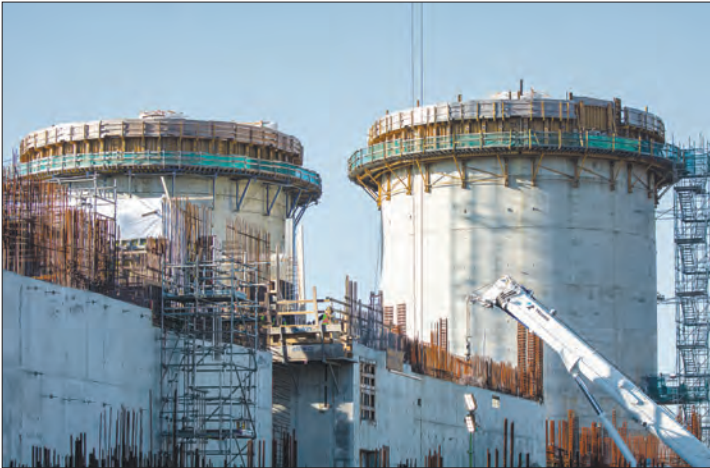
With a new contractor hired, work has ramped up again at the North Shore Wastewater Treatment Plant. NICK LABA / NSN
