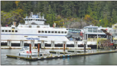
Major upgrades are coming to the Horseshoe Bay ferry terminal over the next several years. PAUL MCGRATH / NSN
