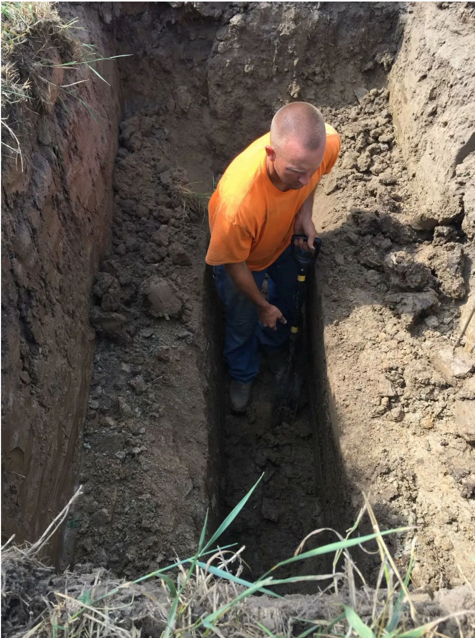
Harold Beach's son, Chris Beach, sets up a trench before laying drainage tile. Beach said drainage tile significantly improved his crop yields. Courtesy: Harold Beach
